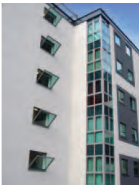
ABOVE Orion Apartments, Navigation St LOCATION: BIRMINGHAM ARCHITECTS: BBLB & JOHN ROCHA CONSULTANTS: HOARE LEA MAIN CONTRACTORS: TAYLOR WOODROW SECO 24 40 ACTUATORS INSTALLED TO BOTTOM HUNG VENTS AS PART OF COMPLETE SMOKE VENT SYSTEM
